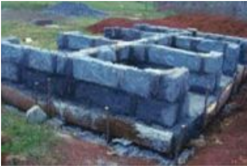
Toilet under construction
