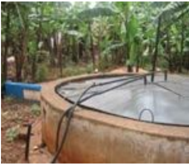
A biogas plant
